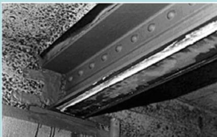
Slattocks Canal Bridge
